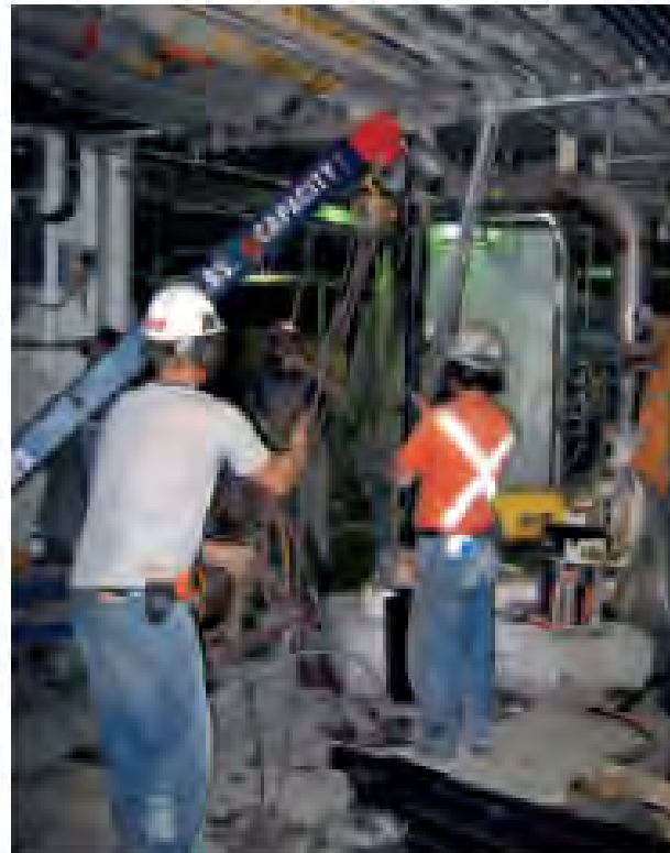
Pile Installation in limited head room
