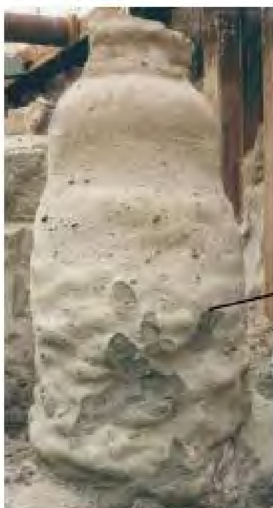
Colunas jet grouting
